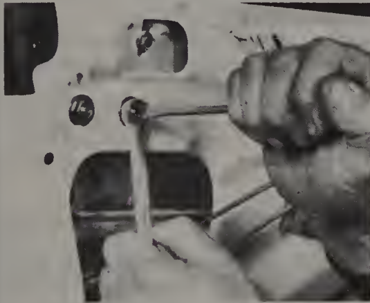
13.36 Upper sash adjusting bolts
