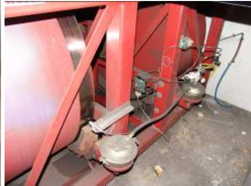
Pic under the floor
