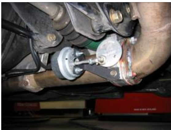
AES System Installed
