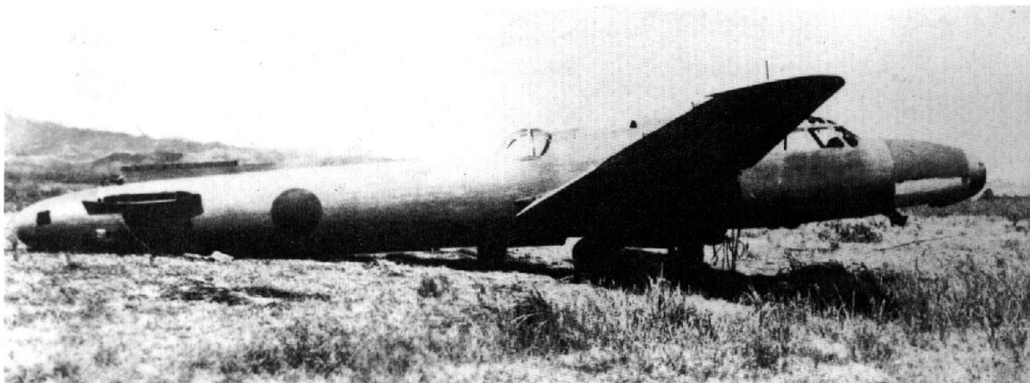
Modified at the Tachikawa Army Air Arsenal in August and September 1944, ten examples of Ki.67-I Special Attack bombers with plywood noses were completed in time for use by the Fugaku (Mt. Fuji) Special Attack Corps in the Philippines Campaign. This one was caught on the ground before it could be used. USAAF.
