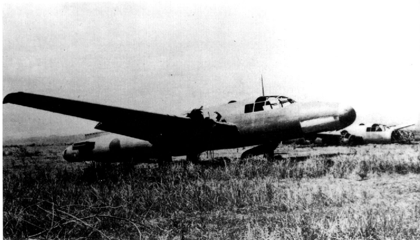
Nose, tail and side gun positions of the Fugaku Corps Ki.67-I suicide bombers were faired over with plywood. Crew was reduced to three men. USAAF.
