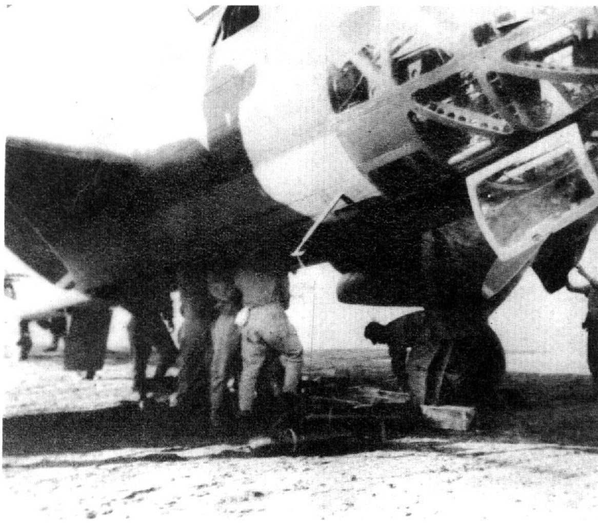
Normal Hiryu bomb load was eight 220 lb. Type 94 or three 551 lb. Type 92 bombs, for a total of around 1,700 pounds. Sekai no Kokuki.
